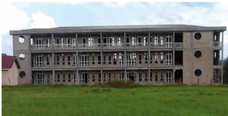
Technical School, visione frontale
